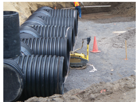
PREPARING THE SOIL FOR HDPE PIPE INSTALLATION
