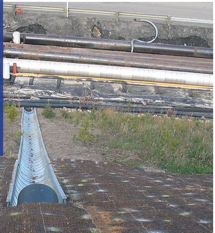
DITCH LINER SUPPORTED BY TIMBER RUNNERS
