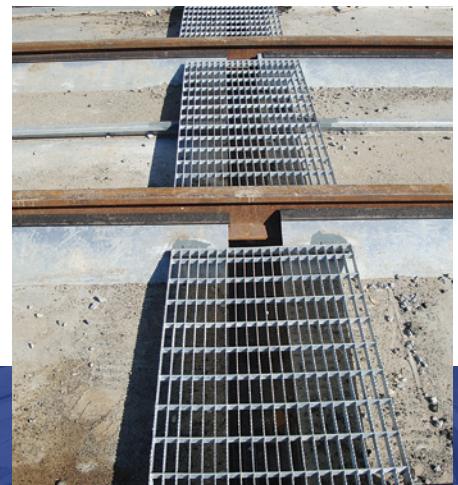
COLLECTOR PAN WALKWAY
