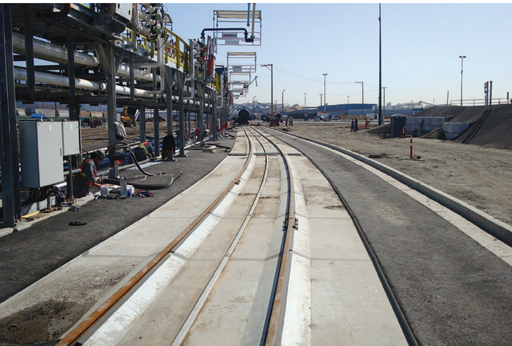
COLLECTOR PANS FLOAT ON TIES MAKING THEM UNAFFECTED BY NORMAL VERTICAL MOVEMENT
