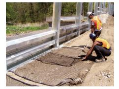
Open-mesh polymer-based geosynthetics-
