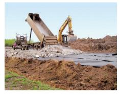
Woven and non-woven geotextiles made from polyester or polypropylene-
