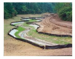
Controls and filters silt-laden runoff during site development and construction-
