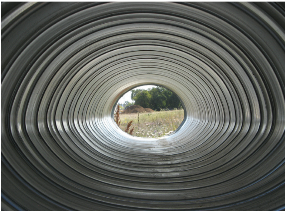
PIPE ARCH SHAPES CAN BE SUPPLIED WHERE THERE IS LOW HEADROOM
