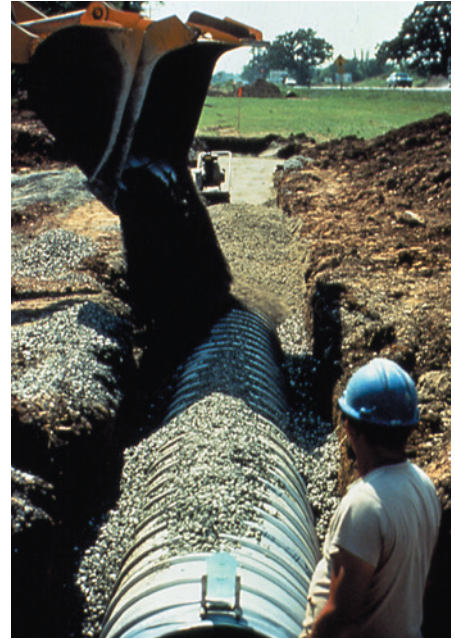
ULTRA FLO STEEL PIPE - BACKFILLING
