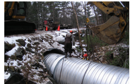
A BAND TYPE COUPLER IS TIGHTENED AROUND PIPE ENDS
