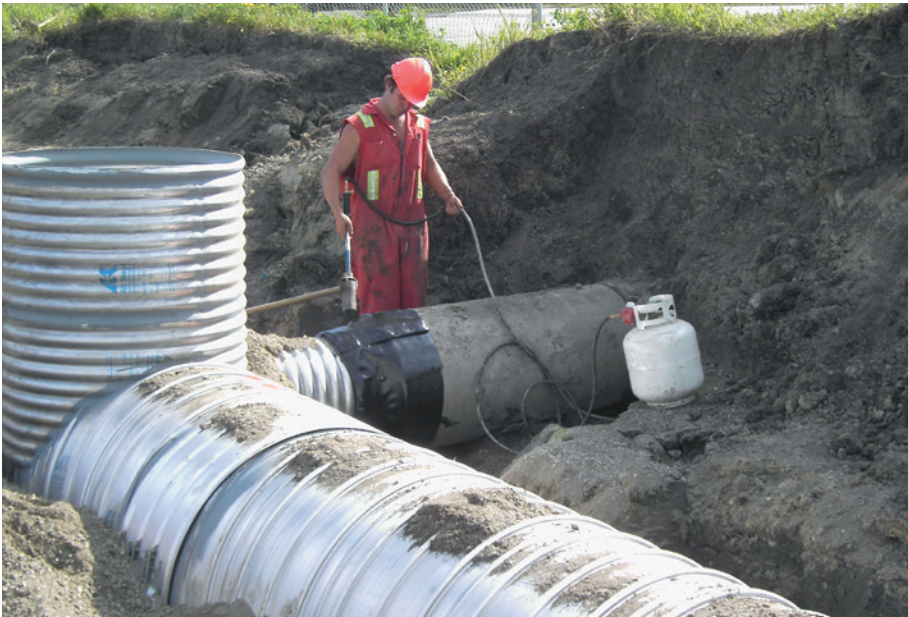
A TEE IS SHOWN COMBINING A STANDARD HEL-COR STUB WITH AN ULTRA FLO STORM SEWER PIPE
