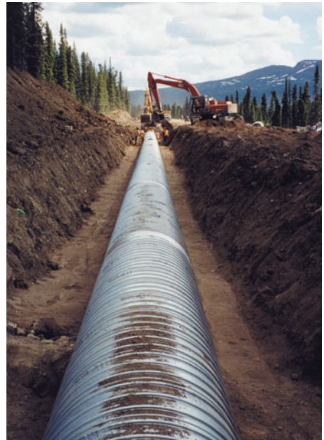
LONG LENGTHS AND POSITIVE JOINTS ASSURE GOOD ALIGNMENT AND LEAK RESISTANT PERFORMANCE
