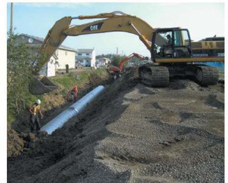
ULTRA FLO PIPE CAN BE INSTALLED IN TIGHT CONSTRUCTION ZONES
