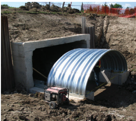
TUNNEL LINER PLATE CAN BE USED TO LINE A VARIETY OF SHAPES, INCLUDING OPEN BOTTOM STRUCTURES
