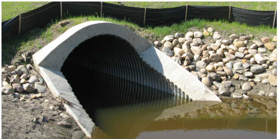
BEVELLED END WITH REINFORCED CONCRETE COLLAR
