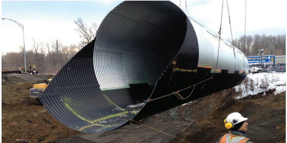
STRATA-CAT POLYMER COATING PROVIDES EXTRA PROTECTION IN AGGRESSIVE ENVIRONMENTS
