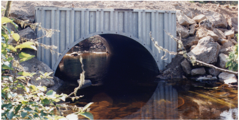
SHEET PILE HEADWALL
