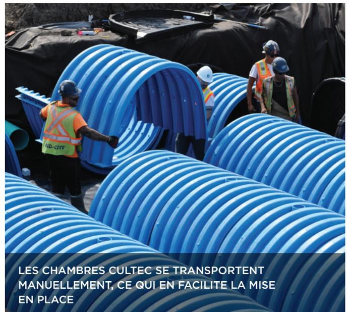
LES CHAMBRES CULTEC SE TRANSPORTENT MANUELLEMENT, CE QUI EN FACILITE LA MISE EN PLACE
