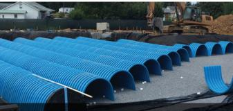
CULTEC'S RECHARGER SERIES ARE HIGHER PROFILE, LARGER CAPACITY CHAMBERS FOR MAXIMIZING STORAGE IN A SMALL FOOTPRINT
