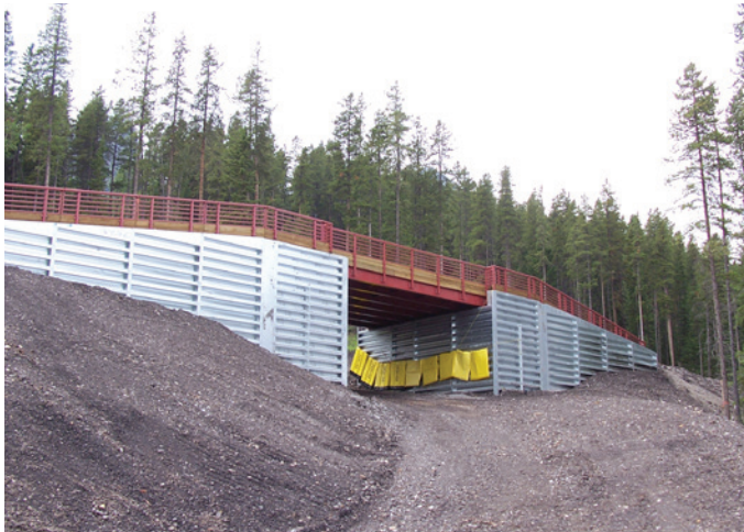
WOOD FACING ENHANCES THE NATURAL APPEARANCE OF THIS BINWALL BRIDGE ABUTMENT
