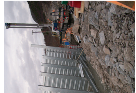
BINWALL CAN BE BOLTED TOGETHER ON SITE OR DELIVERED TO THE JOB SITE PREASSEMBLED
