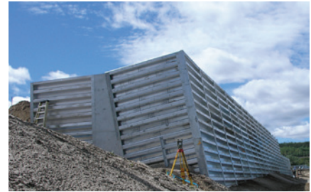
BATTER BINWALL BETTER ACCOMMODATES MINOR GROUND MOVEMENT
