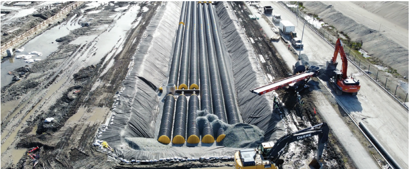
Detention system layout and the placement of gravel surround.
