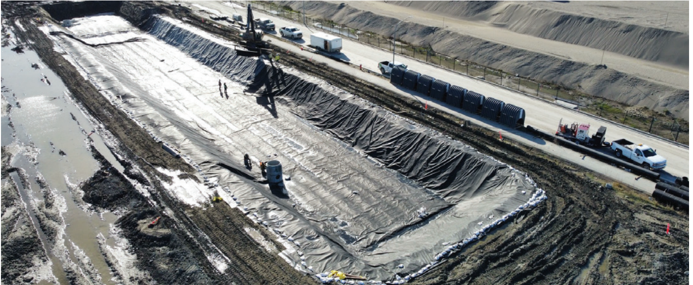
Detention system excavation, geotextile and liner installation.
