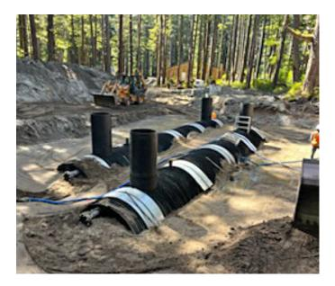
The project was completed in July 2023. The sanitary storage tanks now collect overflow and prevent the discharge of untreated waste into the nearby ocean and waterways.
