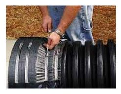
**FIGURE 2:** Dissimilar pipe coupler with rubberized sealing mastic and steel compression bands (*ref. Mar Mac*).
