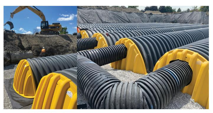
Find out how **HydroStor Stormwater Chambers** can be used on your next project!
